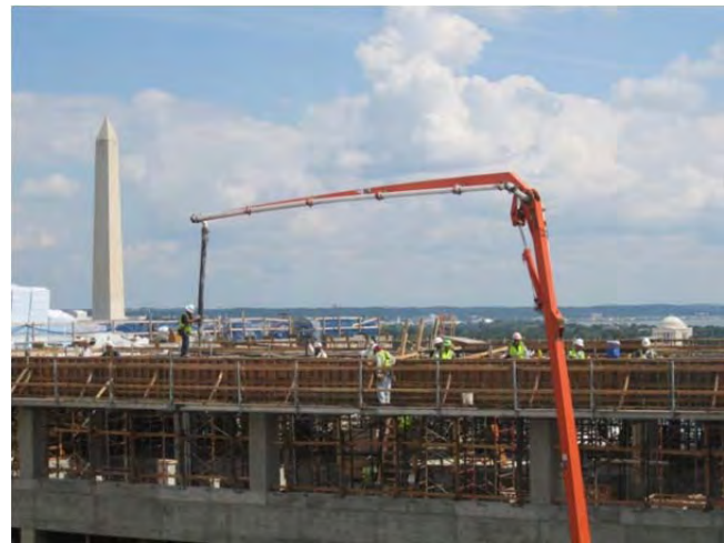
Figure 8: Roof slab of the New Addition – Photo Taken by Ramuel Holgado
