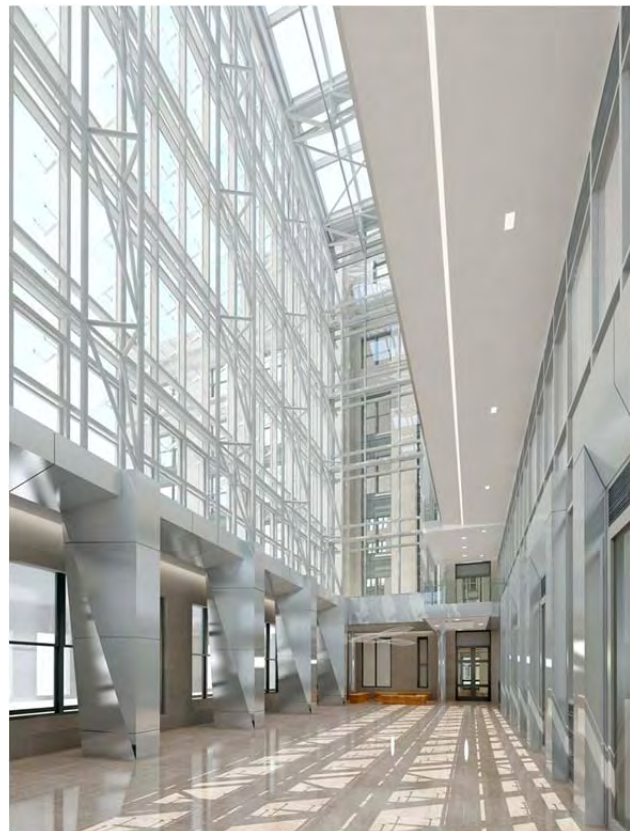
Figure 13: Interior rendering of the atrium showing the curtain wall system – Courtesy of the Whiting-Turner/Walsh Joint Venture
