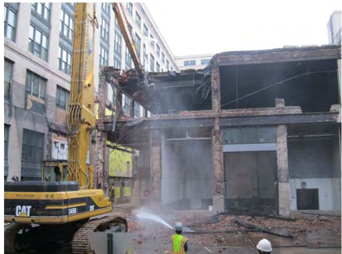
Figure 7: Demolition in the East Courtyard - Courtesy of the Whiting-Turner/Walsh Joint Venture
